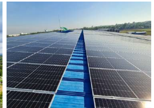
Installation of Solar Panels at HANSAE MYANMAR CO., LTD.
