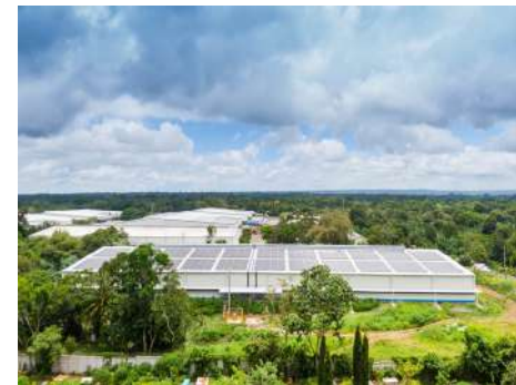
Installation of Solar Panels at HANSAE INTERNATIONAL, S.A.
